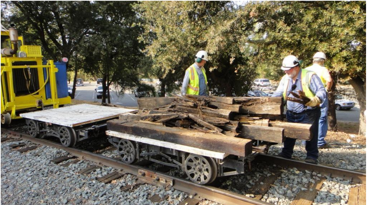
Steve and Frank, along with the rest of the crew, load dead ties we’ve pulled out onto the flat cars
