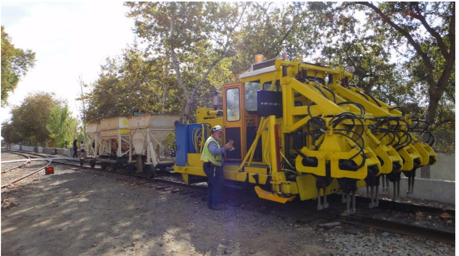
First shake-down cruise complete, Conductor Frank makes the call to Omaha requesting a green light to send the New-old Tamper and hopper-cars back over to the Yards
