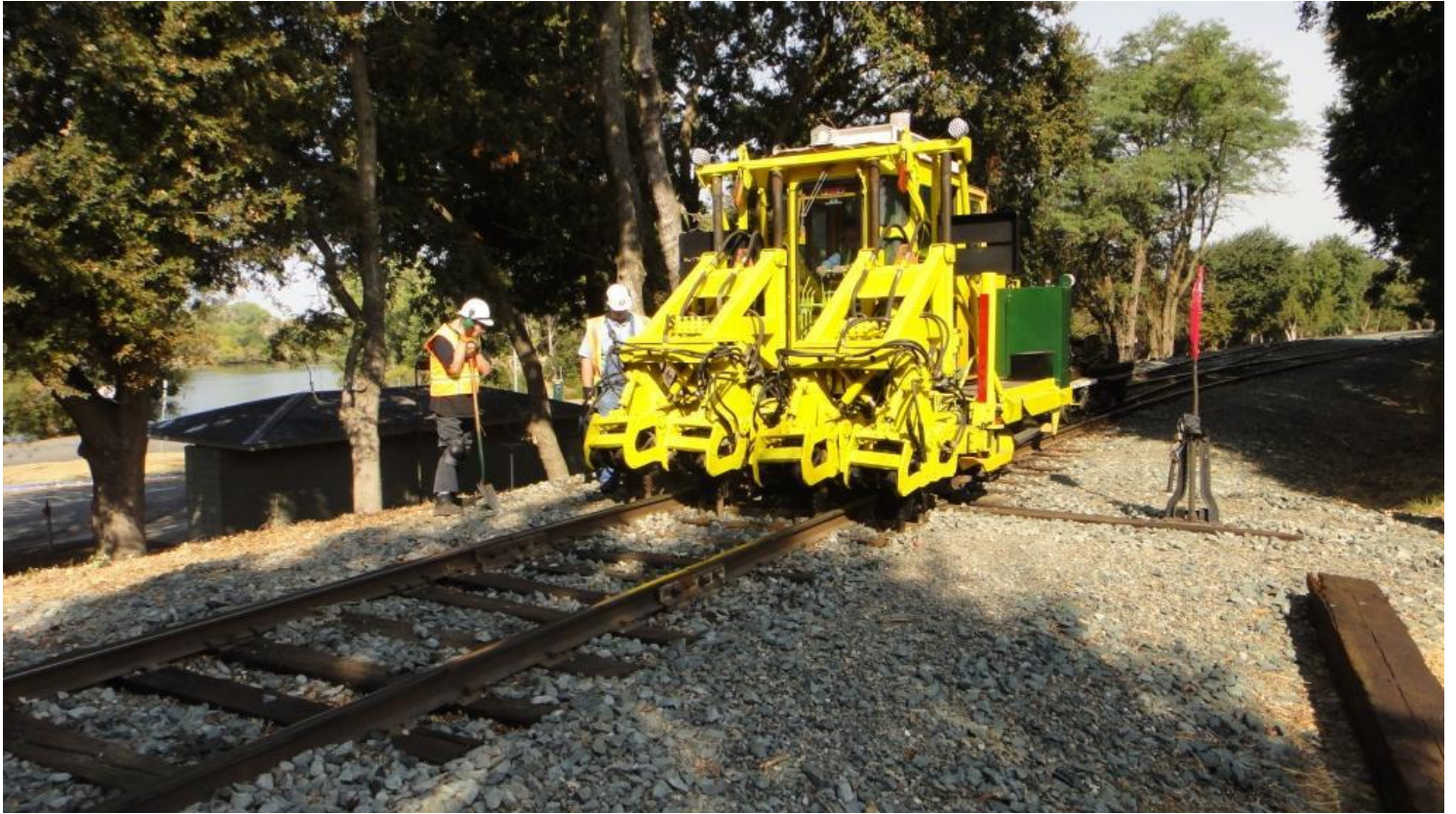
The new-old tamper “shaking-up” the ties to the north of the points at Switch 16
